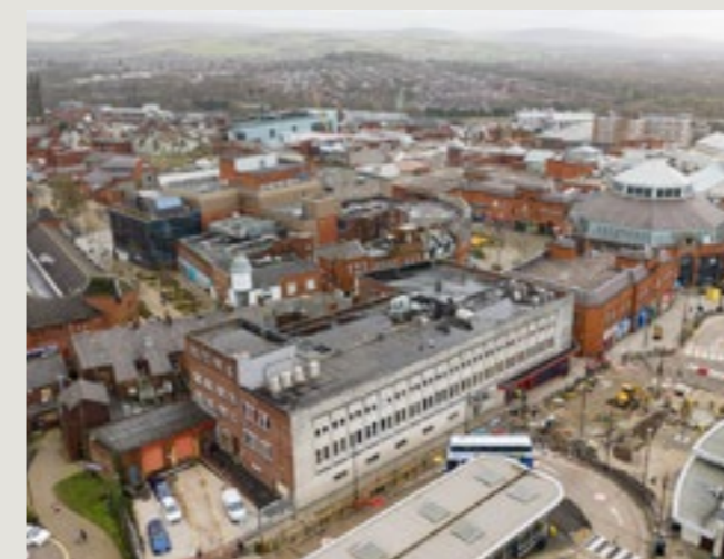
→ FIGURE 6.17 HENSHAW HOUSE
