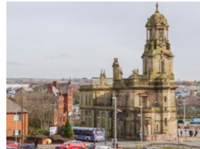
→ FIGURE 5.16 FORMER NATWEST BANK, OLDHAM MUMPS IMAGE CREDIT: PLANIT (FIONA FINCHETT)
