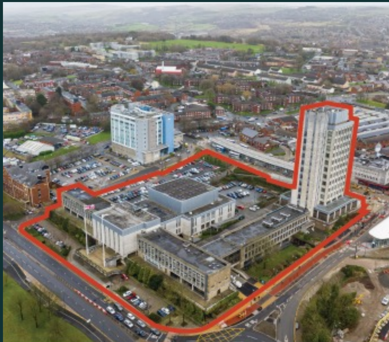
→ FIG. C3 – AERIAL VIEW OF THE CIVIC CENTRE AND QUEEN ELIZABETH HALL
