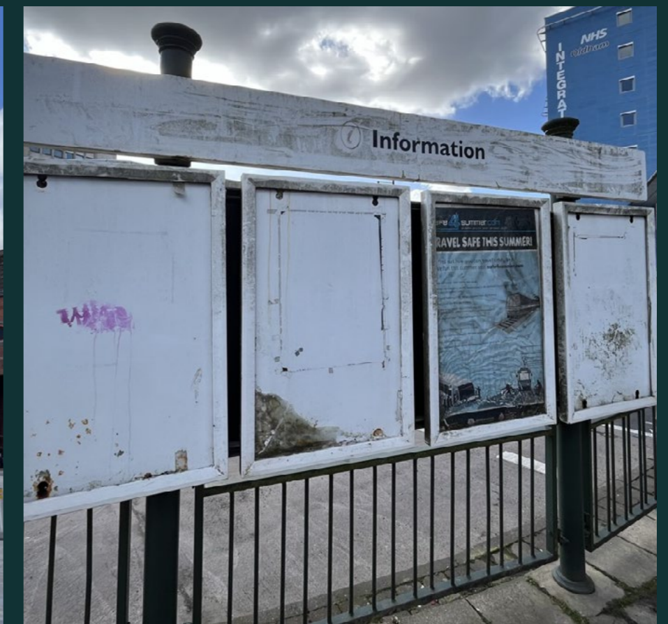
→ FIG. B11 - EXISTING SIGNAGE AND WAYFINDING. FIGURE CREDIT: PLANIT
