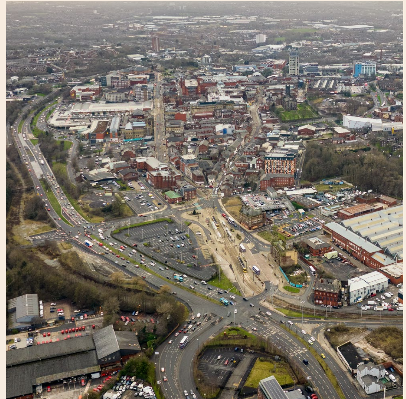
→ FIG. C7 – OLDHAM TOWN CENTRE
